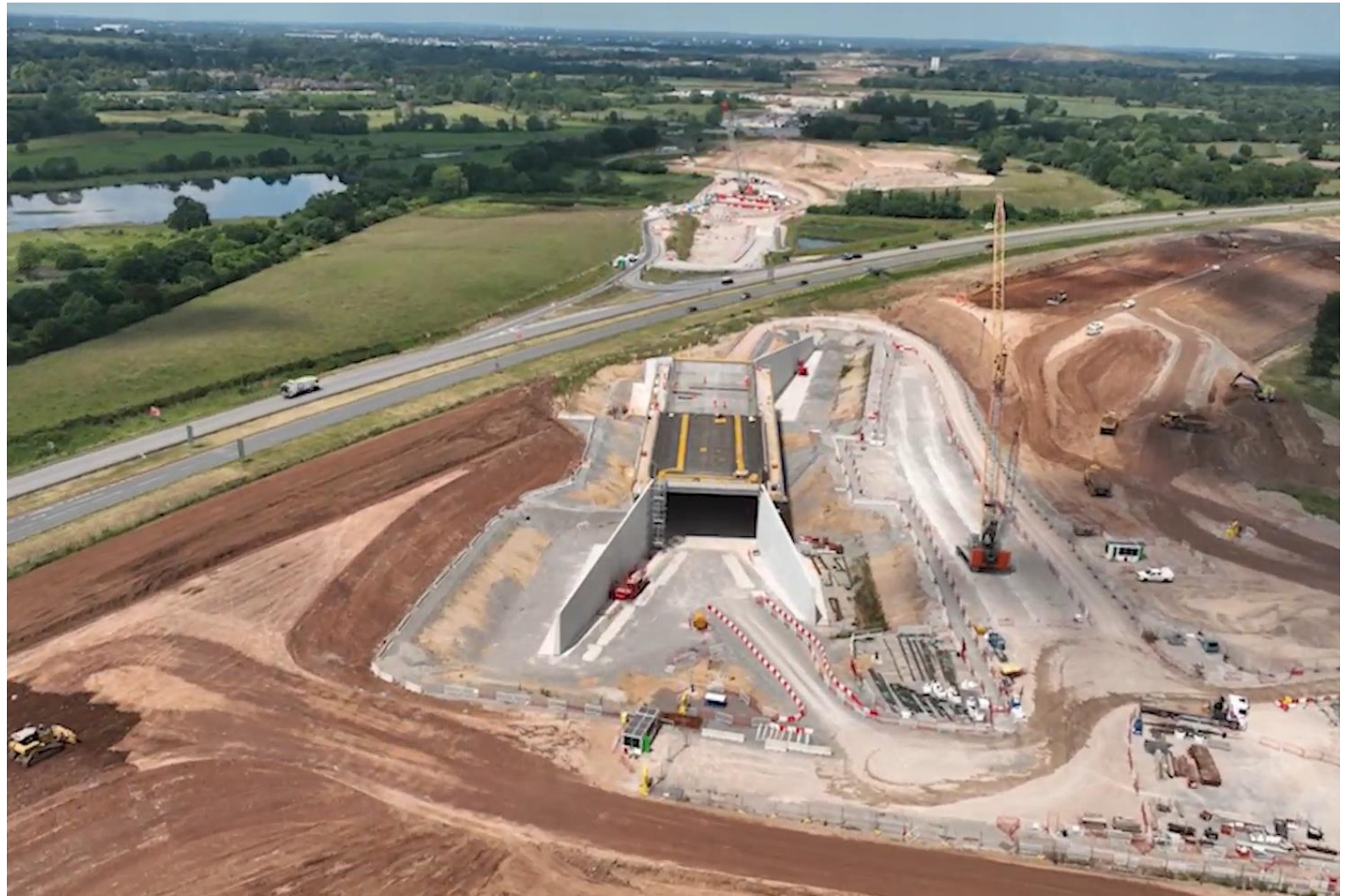
A452 Kenilworth Road Overbridge being constructed off-line
